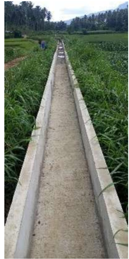
Udaxeragama Canal which will benefit around 750 people
